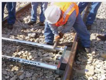
Inserting the MTW into the track and expanding the system via the threaded support poles
