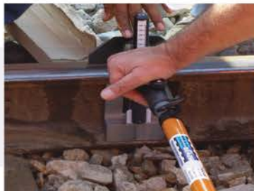
Measuring the height to determine the shim size
