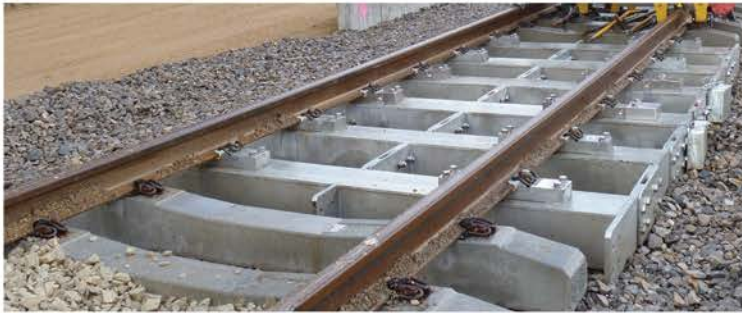
Installation of INFINITY 'LS' weighing system in straight track
