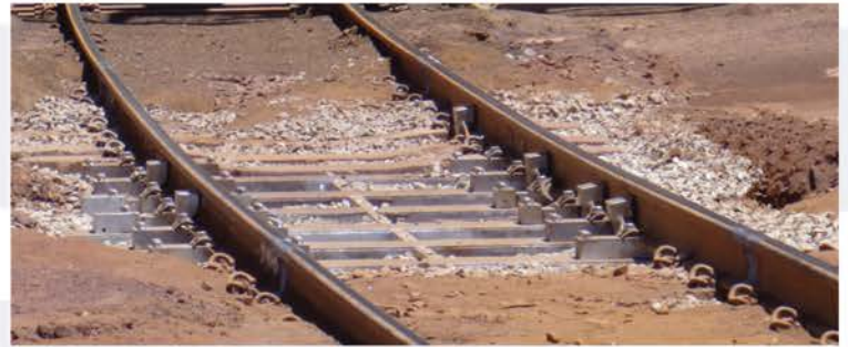
Installation of INFINITY 'LS' weighing system in curved track
